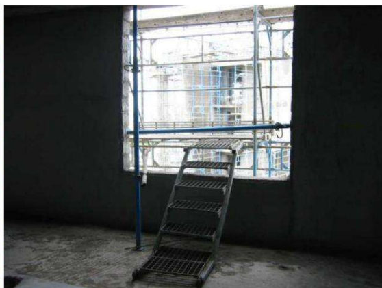
Proper Access to workplatform
