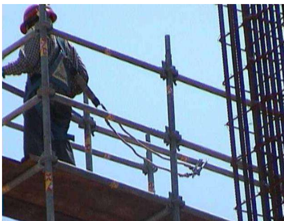
Full body harness with double lanyard
