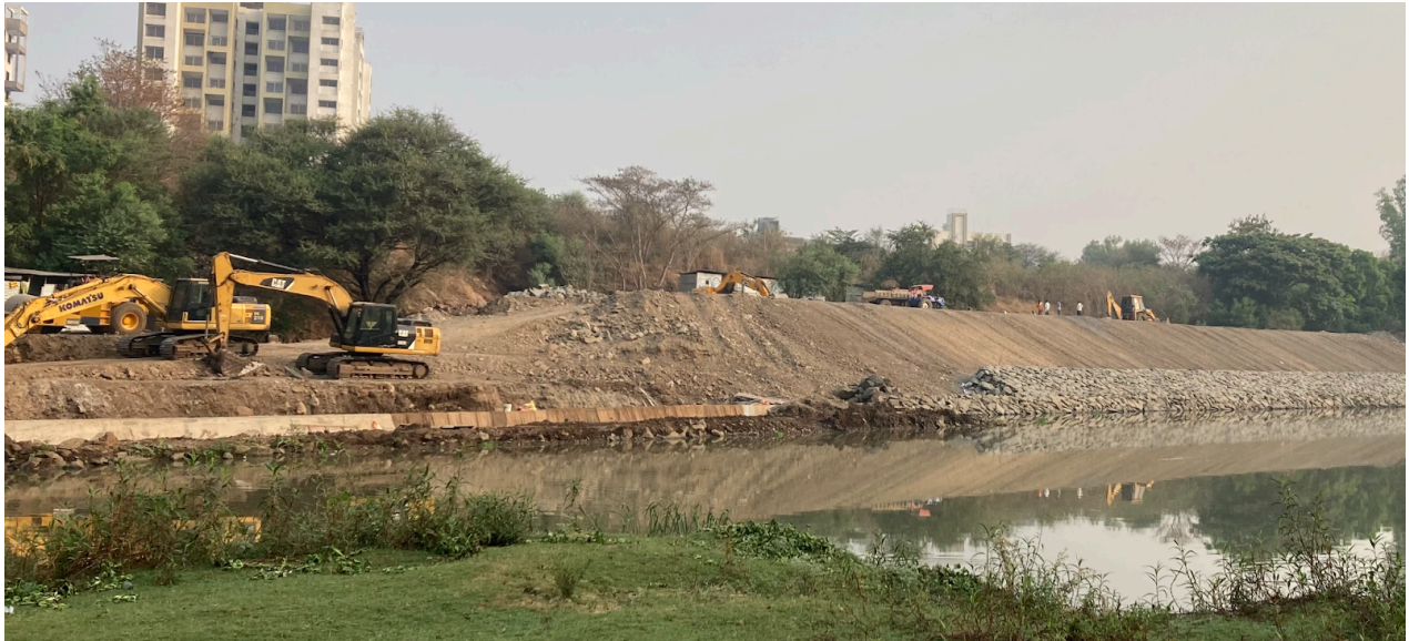
Large-scale construction activity at the Mula-Ramnadi confluence (Photo by Banerjee, 03/04/2025).
